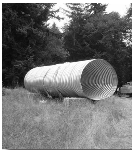
The new culvert is 8 feet wide x 20 feet long. The original concrete pipe was only 16 inches wide and 6 feet long.
